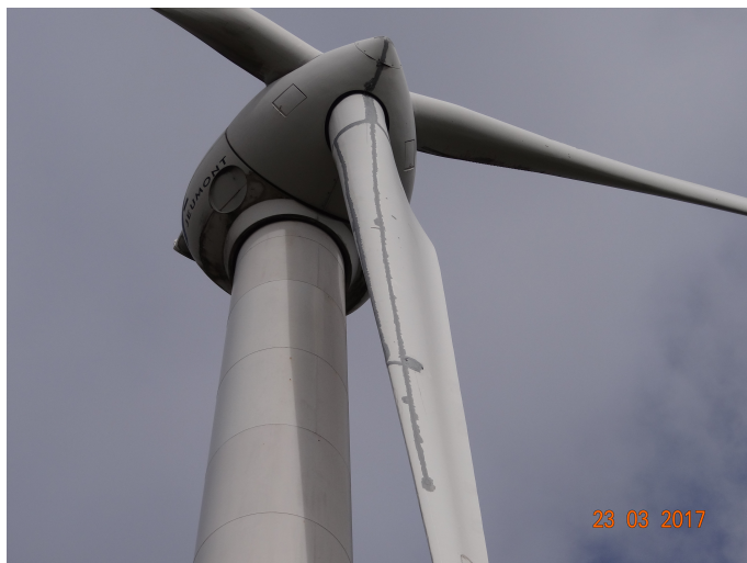
Figure 7. Photo of the pressure side of the wind blade after instrumentation
