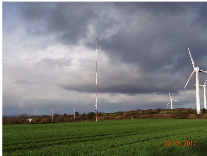
Figure 5. Photo of the met mast after its installation
