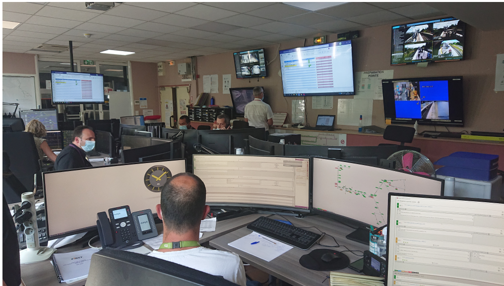
Figure 7: Control room D and R lines, Paris, France.
